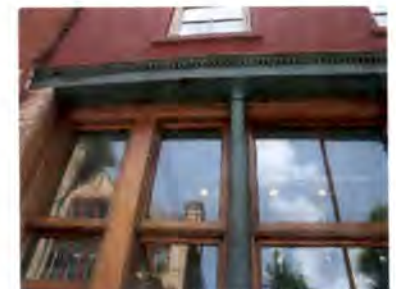
The metal cornice and columns on this storefront are unique features that should be preserved.
