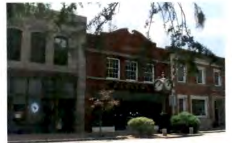
Baxter's unique curved coping creates visual interest when compared to the parapets and cornice lines of surrounding buildings.
