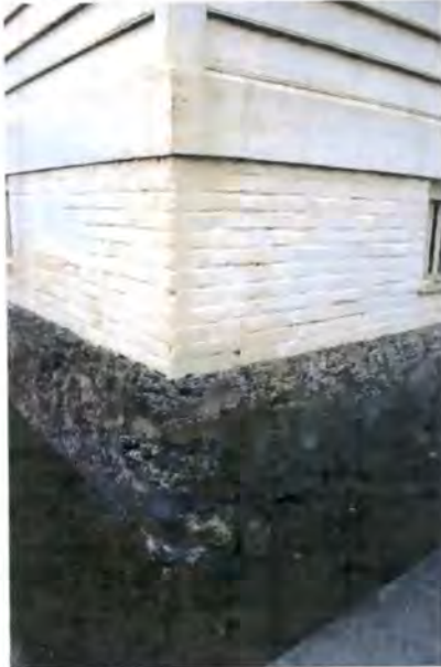
An example of a marl and brick foundation.
