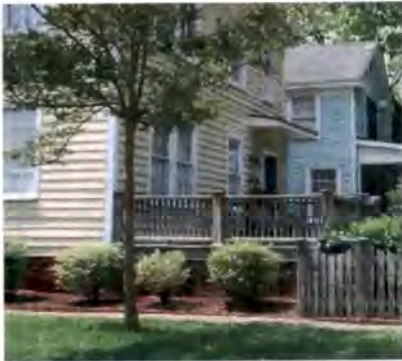
The deck on this house is located in a Secondary AVC screened by shrubbery, and it has a foundation similar to the main structure.
