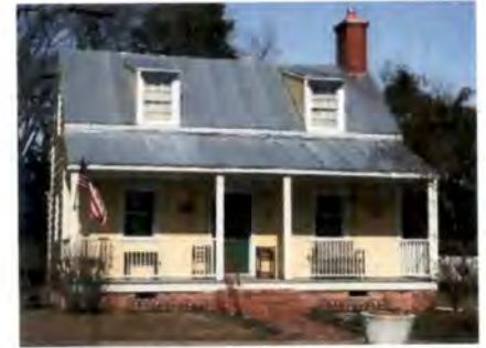
Standing seam metal is a common roof material in the historic districts resulting from reduced insurance rates following the Great Fire of 1922.
