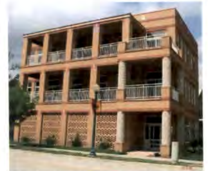
This building is located in the transitional edge between dense fabric and tight weave development patterns. The use of a modern blonde brick and patterned masonry is appropriate for this infill construction.
