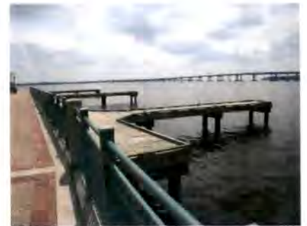
The piers and bulkheads at the waterfront park are consistent with the design guidelines. They are built of wood and concrete, and do not diminish scenic views.
