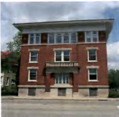
The wide cornice, overhang, and brackets add character to this building.
