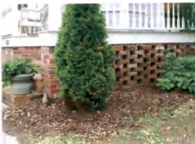
An example of brick lattice.
