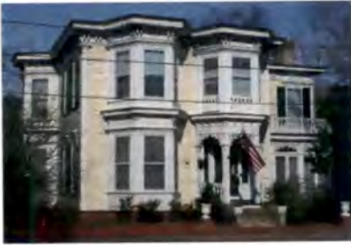
A bracketed cornice, paneled friezes, ornate window surrounds, and embellished porch are some of the wood elements evident on this house.
