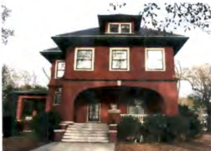
This house in the Riverside Historic District has a brick masonry veneer at the first floor and wood shingle siding at the second floor.
