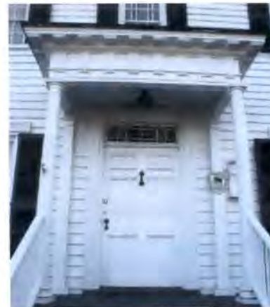
The door, transom, molded surround, corner blocks, pilasters, columns, entablature, flat roof, and stair combine to compose this fine entrance.
