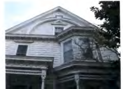
This house displays clapboard, decorative shingles and an abundance of decorative wooden elements that contribute to the character of its fenestration.
