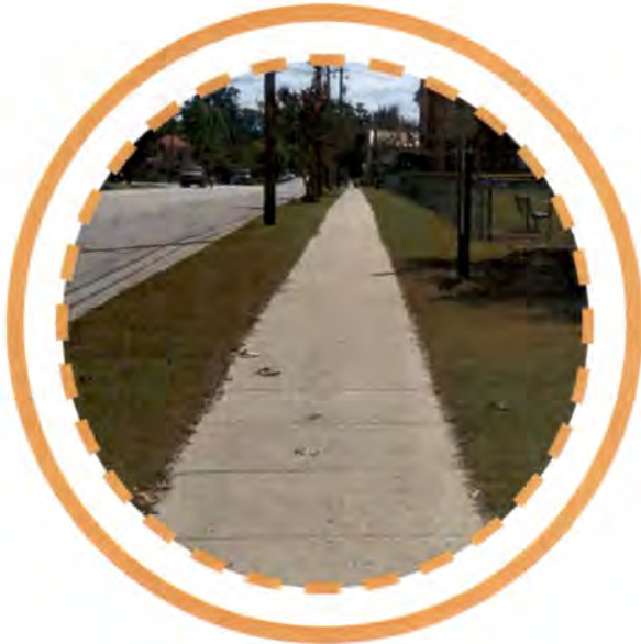
Sidewalks should be physically separated from the roadway by an unpaved buffer separation, barrier or curb edge.
