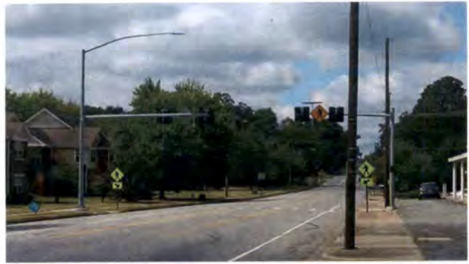
Pedestrian Hybrid Beacons stop automobile traffic for bicyclists and pedestrians wishing to cross a high traffic volume/high speed roadway.
