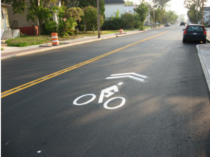
A sharrow image depicts a shared-lane marking indicating that motorists and bicyclists are sharing the lane.
